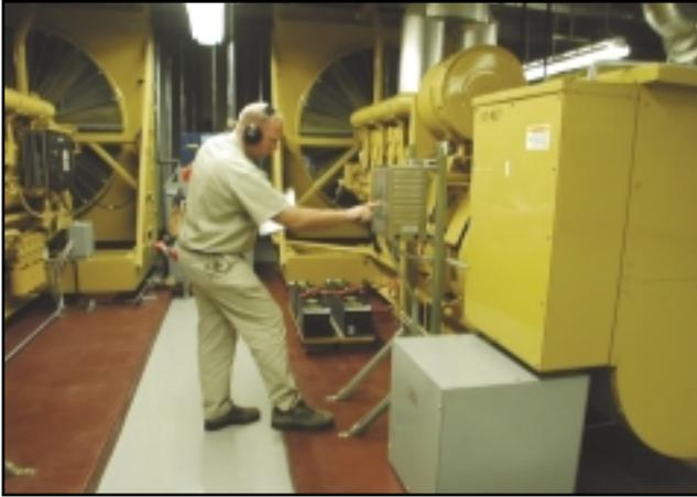
**VENETIAN POWER MANAGEMENT STAFF PERFORM PERIODIC CHECKS OF BACKUP DIESEL ELECTRIC GENERATORS, WHICH CAN PROVIDE UP TO 10 MEGAWATTS OF POWER FOR THE HOTEL.**
